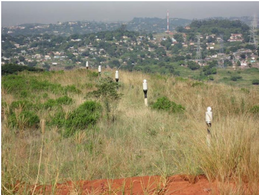
Plate 4: The gas system: the whirly birds were all working at the time of the audit.
