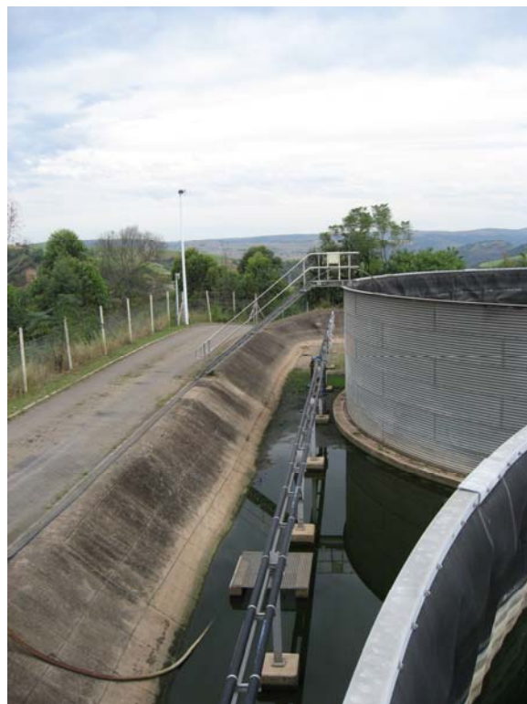
Plate 6: View from the Top of One of the Leachate Storage Tanks above the Offices: the liquid in the bunded area is direct rainfall and run off from the road.
