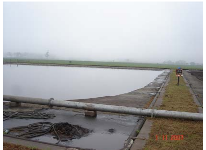
North Slimes Dam: In operation
