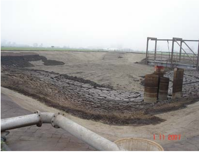
South Slimes Dam: Dry sludge being removed
