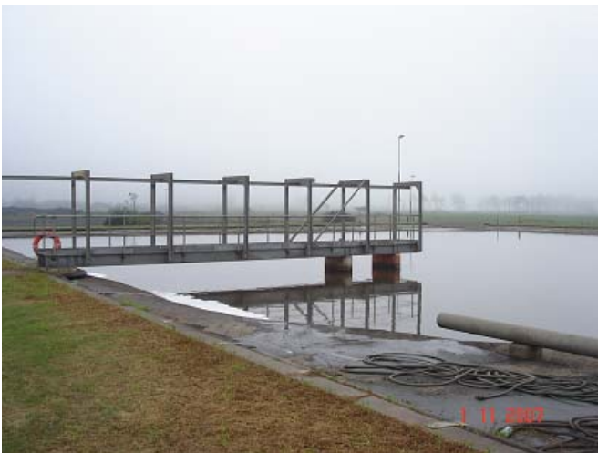
North Slimes Dam: In operation
