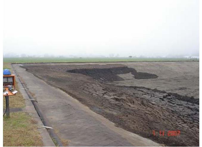
South Slimes Dam: Dry sludge being removed
