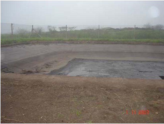
Emergency Overflow Dam
