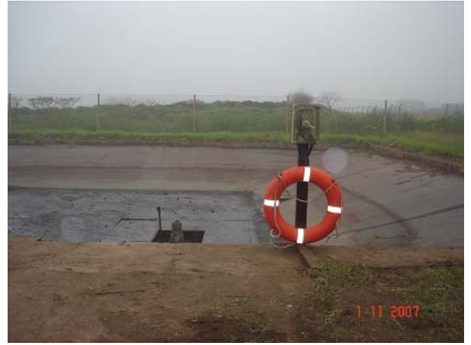
Emergency Overflow Dam
